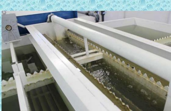
REFERENCE 3 Supplying the Jirásek swimming pool in Náchod with service water Source: Radechovka stream Technology: two-stage water treatment Output Q = 2 x 20 m3/h The output of the water treatment plant is water complying with the Regulation of the Ministry of Health of the Czech Republic No. 238/2011 Coll.
