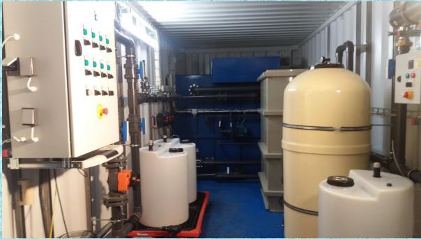
REFERENCE 2 Surface water pre-treatment plant for the Přerov Swimming Complex Source: Strhanec stream Technology: two-stage water treatment Output: Q = 18 m3/h The output of the water treatment plant is water complying with the Regulation of the Ministry of Health of the Czech Republic No. 238/2011 Coll.
